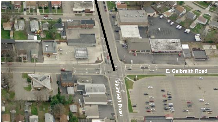
Existing Galbraith Road and Plainfield Road Intersection
